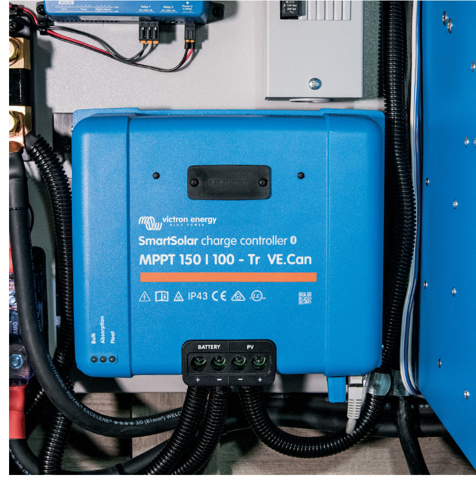
100 amp Victron MPPT Solar Charge Controller
