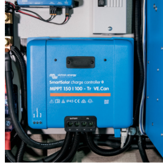
100 amp Victron MPPT Solar Charge Controller
