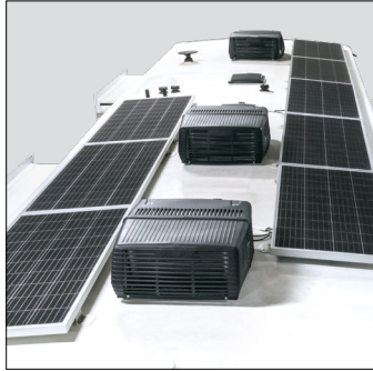
(8) 220W solar panels = 1,760 Watts of solar power
