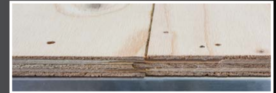
5/8-INCH TONGUE AND GROOVE PLYWOOD floor decking.
