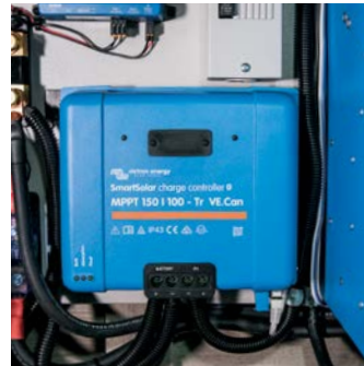
100 amp Victron MPPT Solar Charge Controller
